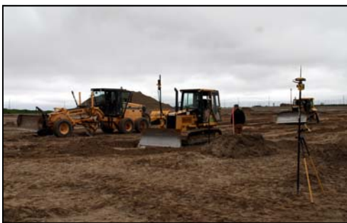
Operators get first hand experience using Topcon's latest machine control technology.
